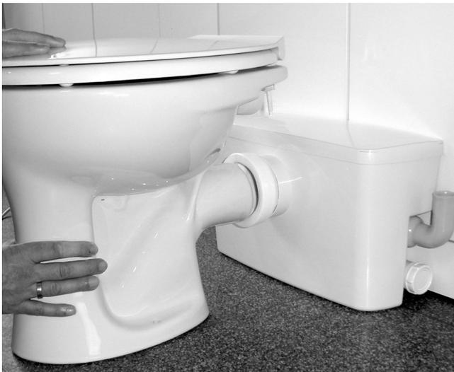
(Pic 1) Place the toilet in front of the unit and push the WC-spigott into the socket of the box. Please make sure that the front of the tank will not be pressed in.
